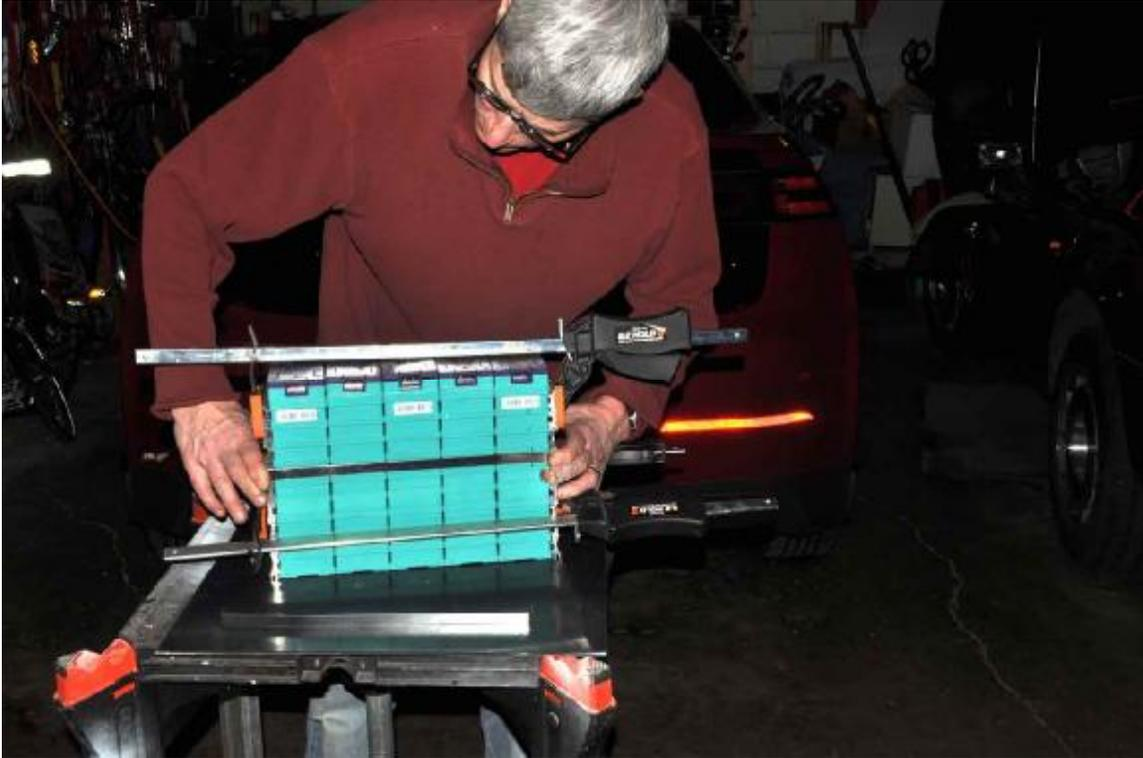
Chris comes by to check on my work. Each strap must be drilled out exactly the same, otherwise the pressure on the cells will not be equal top to bottom.
